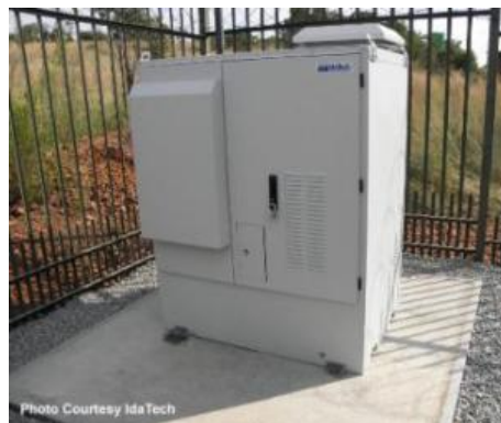
Figure 2: IdaTech system powered by Ballard fuel cell stacks
