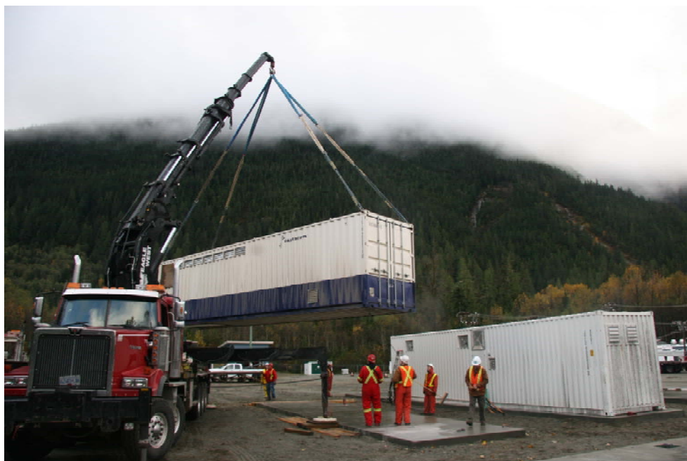
Figure 2: Renewable power system at Bella Coola, British Columbia, Canada.
