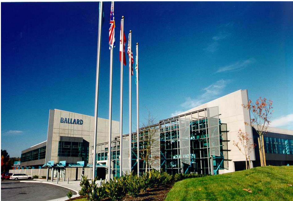
Ballard's HQ facility in Burnaby, Canada. Source: www.ballard.com
